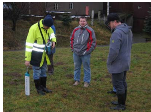
Searching the exact position of the cable with a cable- finder
